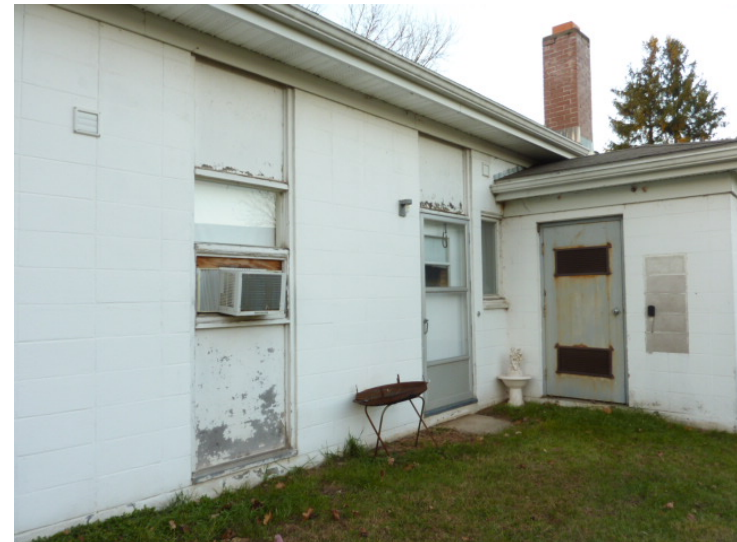
8. Typical failing paint on wood panels and CMU and typical rusting door at Mechanical Room.
