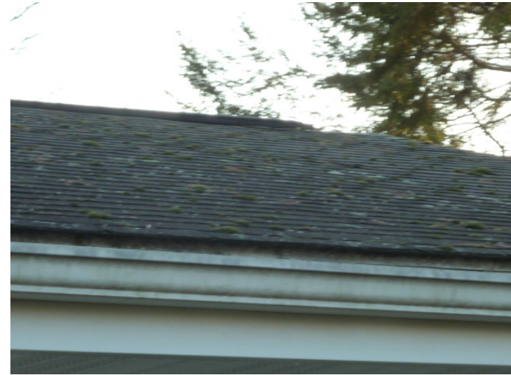
10. Typical asphalt shingles with organic growth and warped shingles.
