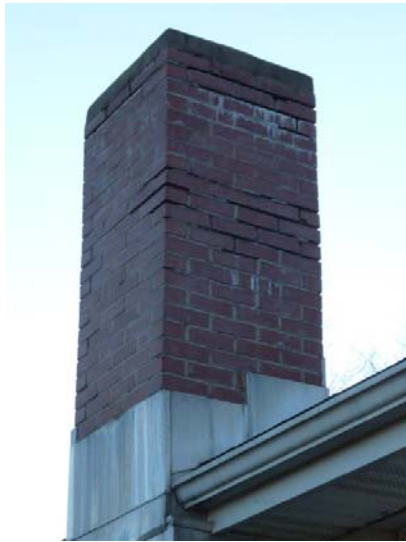
9. Typical open joints at boiler room chimneys.
