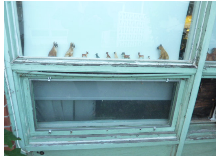
6. Typical deteriorated window at Phase 1 and Phase 2 buildings.
