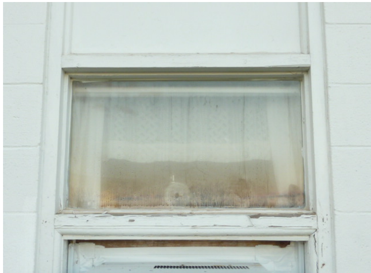
11. Typical failed seals at insulated glass site-wide.
