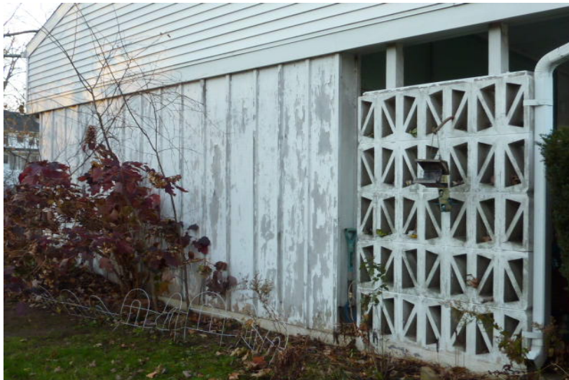
7. Typical failing paint on vertical wood siding and CMU.
